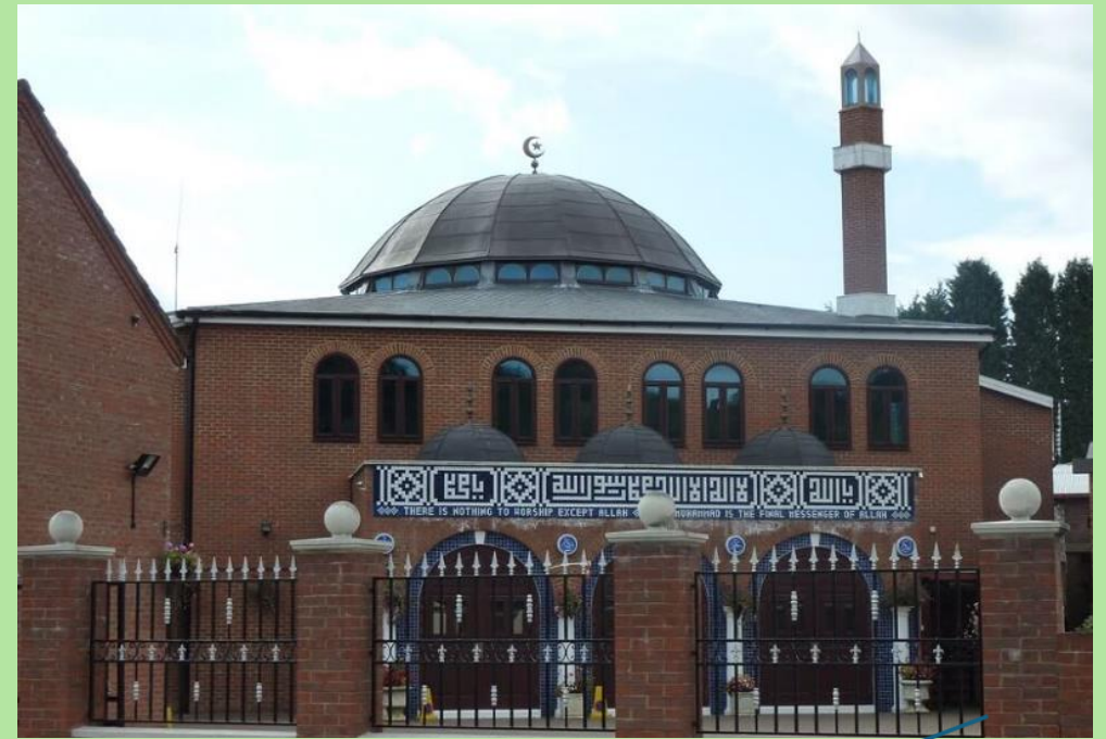
Chesham Mosque, Chesham.
